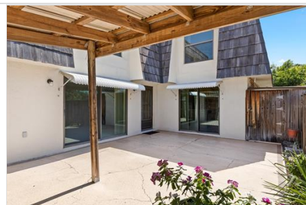
2nd view of Fenced in Patio
